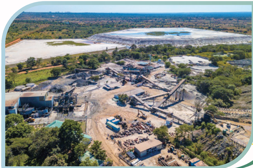
Chibuluma South Mine - Processing Plant Chibuluma南礦場 - 選礦廠
