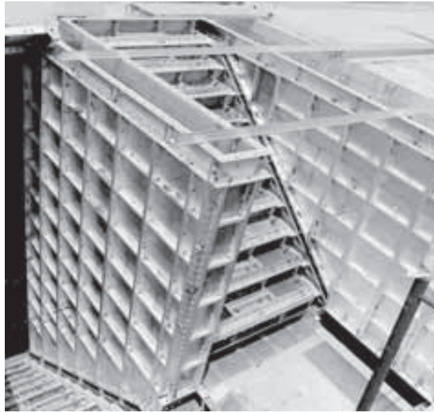
Aluminium formwork for wall and staircase
