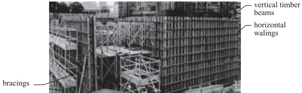
Timber wall formwork
