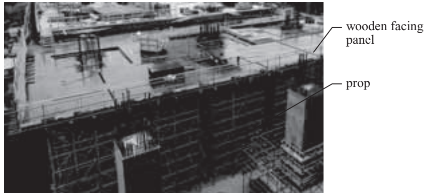
Timber slab formwork
